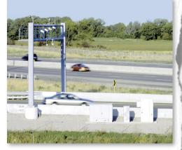
The ETR technology allows motorists to pass through toll routes without stopping or even opening a window. To make this happen, each highway entry and exit point is equipped with a gantry.
